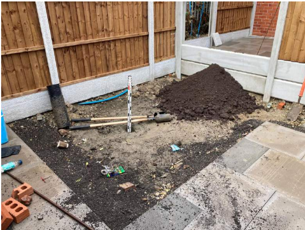
Photograph 4 View of Plot 3 rear garden showing location of VP02 with topsoil stockpiled prior to emplacement.
