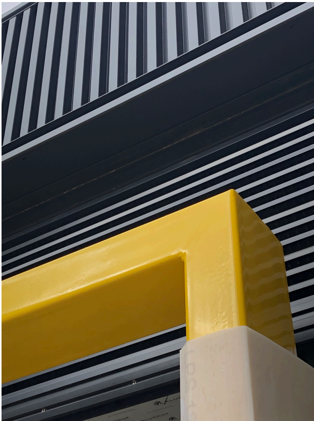
close up photograph from site inspection
