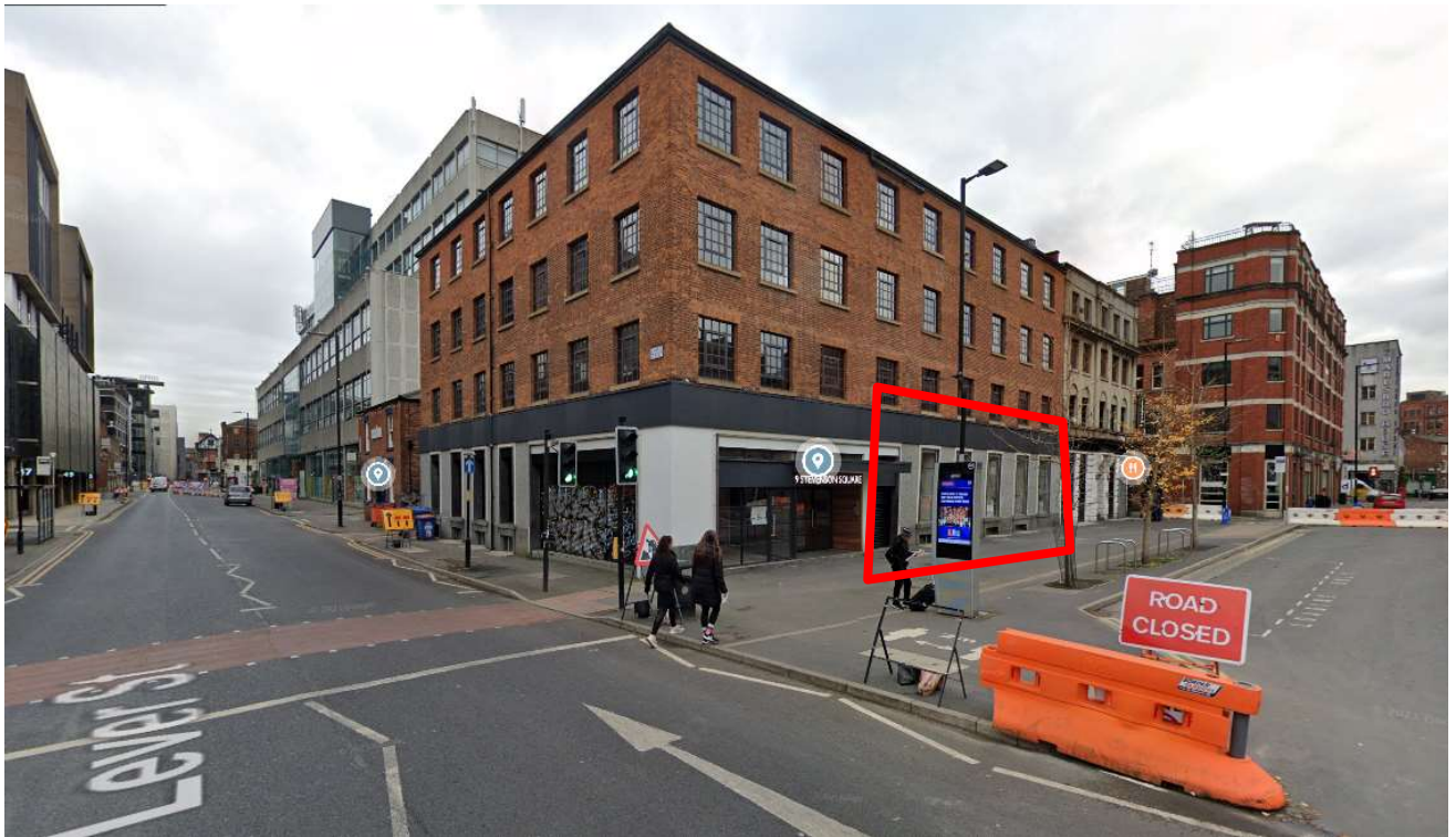
Photo 1. Application site, with the ground floor unit outlined in red. Source: Google maps.
