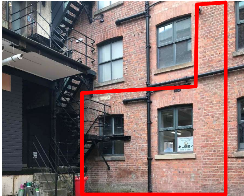
Figure 2-1 Photograph of the rear courtyard elevation showing approximate location of proposed ventilation equipment in red.
