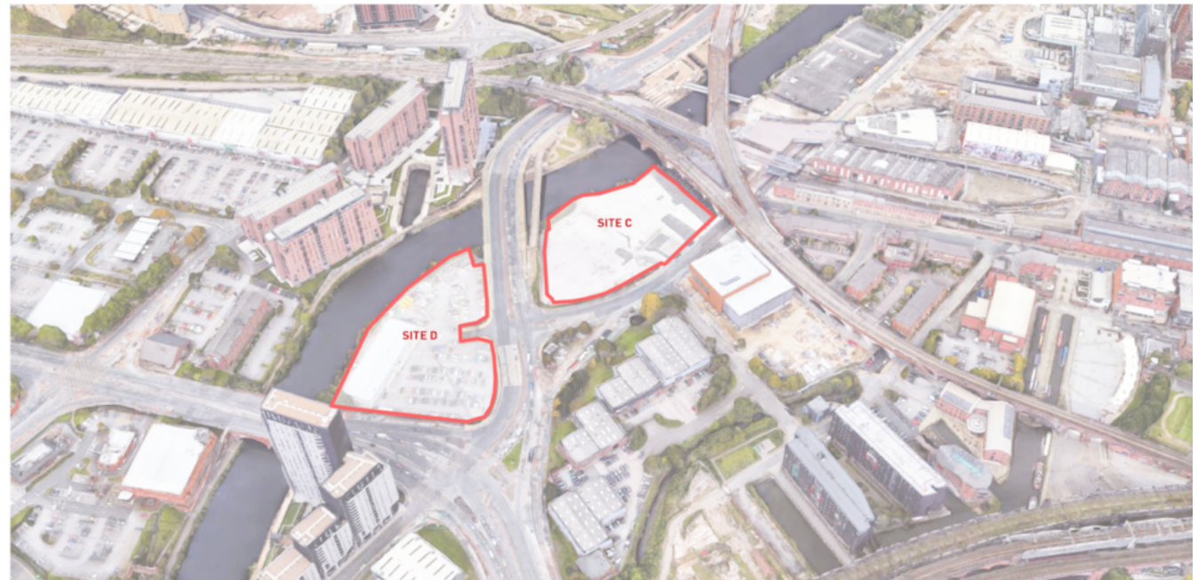
AERIAL VIEW - LOOKING NORTH
