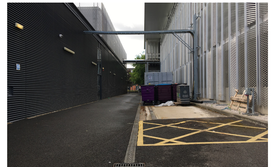
6. The service yard between the Energy Centre and Multi Storey Car Park
