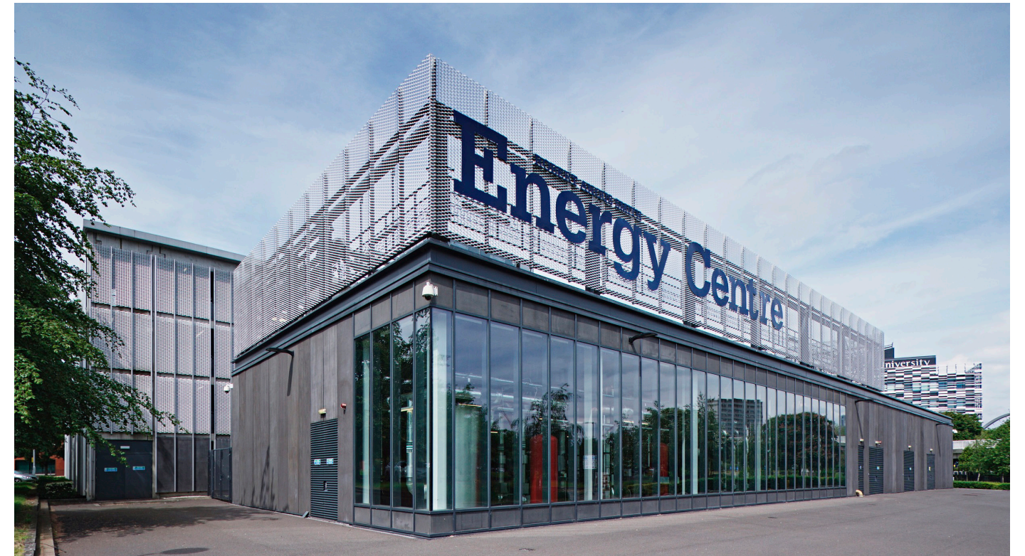
The Energy Centre and Mutli Storey Car Park
