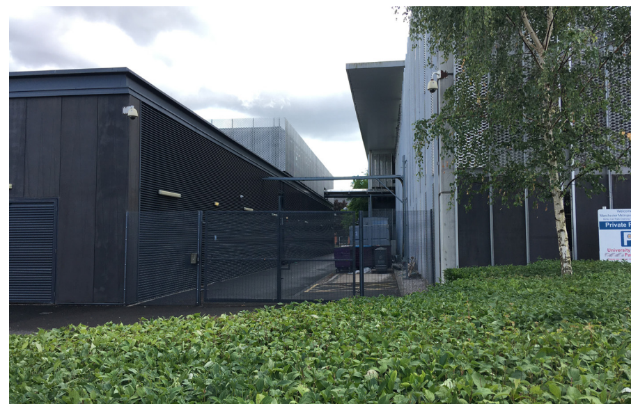
5. View of the exisitng service yard enclosure
