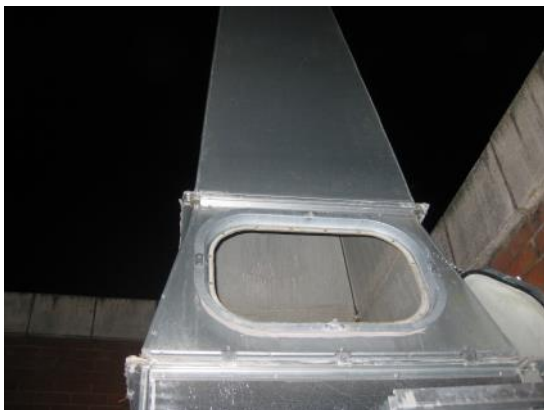
69. DISCHARGE TO ATMOSPHERE PRE CLEAN
