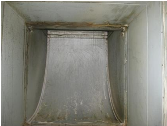
45. ACCESS TO RISER ON 1ST FLOOR PRE CLEAN
