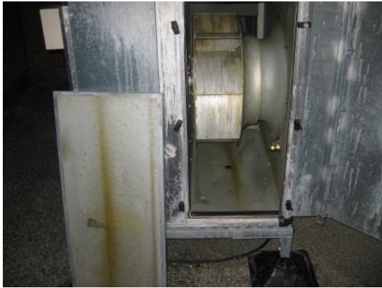
61. DISCHARGE FROM FAN TOWARD TURN TO SOUND ATTENUATOR PRE CLEAN
