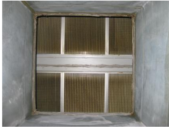
55. DISCHARGE FROM ECOLOGY UNIT PRE CLEAN 56. POST CLEAN
