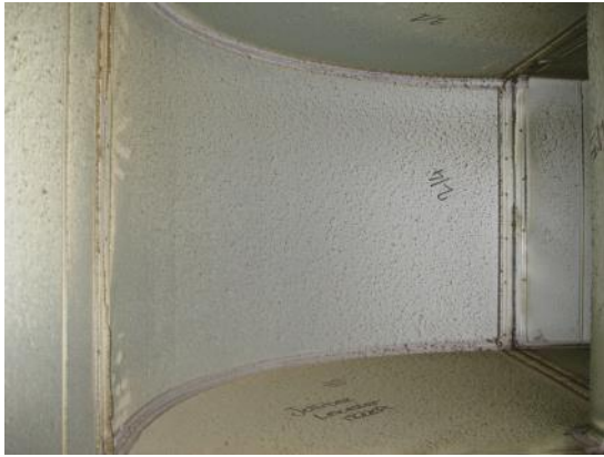
43. BASE OF RISER TO ROOF PLANT SPACE PRE CLEAN
