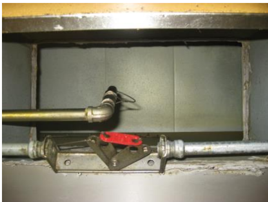
33. TYPICAL SPIGOT TO THE HEADER ABOVE PRE CLEAN
