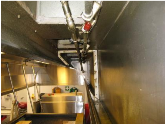
31. TYPICAL SPIGOT TO THE HEADER ABOVE PRE CLEAN
