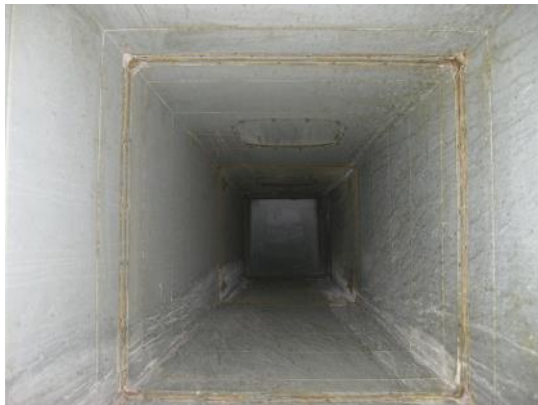
51. TOP OF THE RISER AT ROOF PLANT SPACE LEVEL PRE CLEAN
