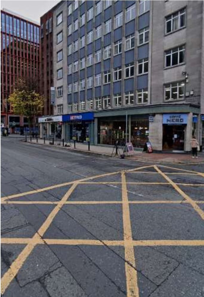
Figure 6: Photo taken from corner of 186 Deansgate facing the application site
