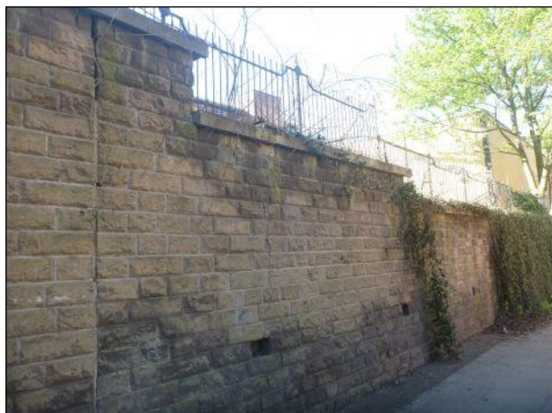
Photo 3: Wall at north-western site boundary
