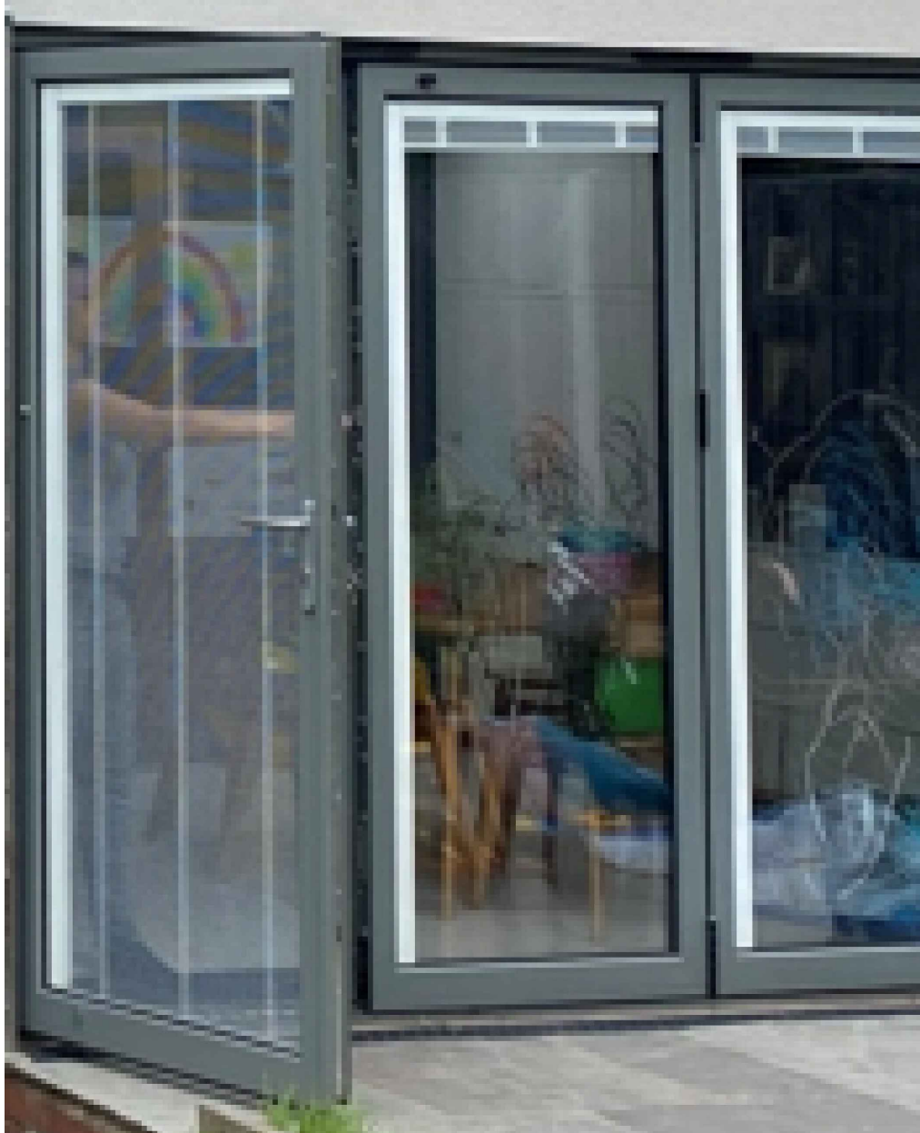
6 New doubled glazed window fittings in RAL colour to match existing bi-fold doors to rear elevation
