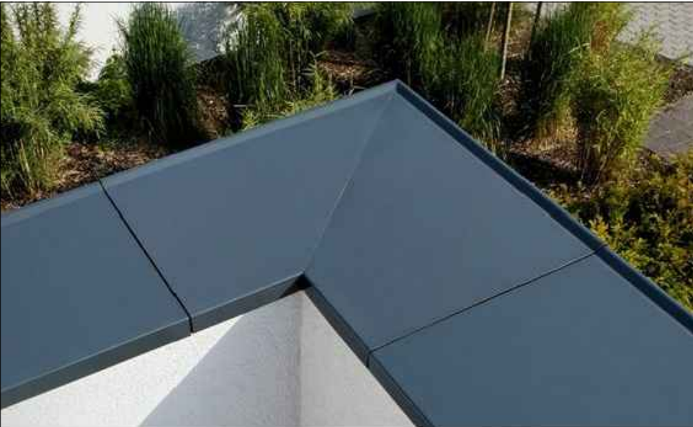
4 New aluminium pressure fixed coping to replace existing artstone fixtures
